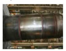
**8. Steam can bypass bolts.** Large bolts inserted into the holes are used to tightly secure the large horizontal joint flange in this high-pressure cylinder. The bolt holes are places where a steam jet leak can form due to cylinder deformation and changing duct pressures. Courtesy: Ahwaz Power Generation Management Co.
